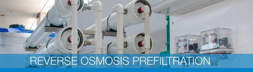
Reverse Osmosis is a water treatment process that removes dissolved contaminants from water by using pressure to force water molecules through a semipermeable membrane. RO water has a wide variety of uses ranging from hospitals and pharmaceutical production to food and beverage and wastewater treatment. In order to ensure that RO membranes continue to operate at their optimum level, incoming water must be prefiltered prior to entering the reverse osmosis system.
